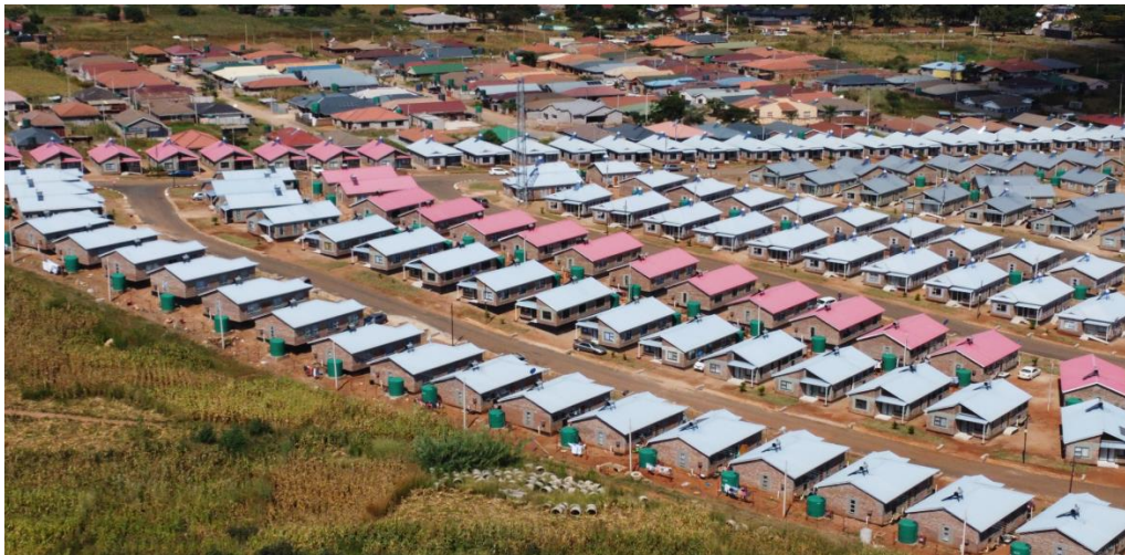
Kuwadzana FBC Housing Project
